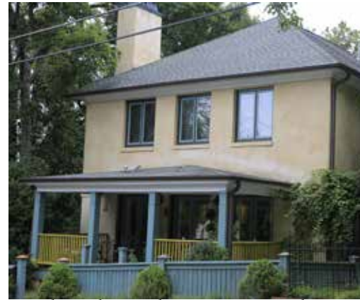
226 Elm St has modern casement windows
