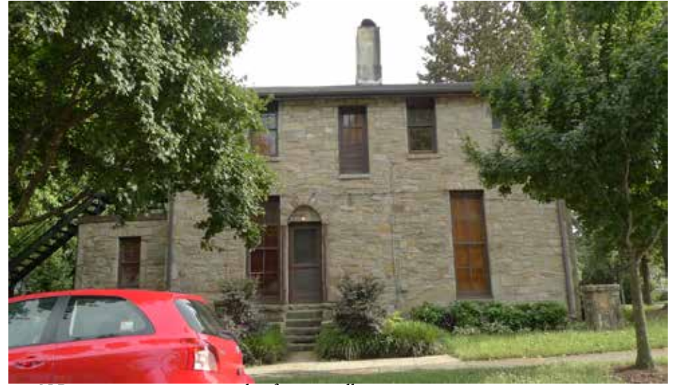
426 N Person street is an example of stone wall construction
