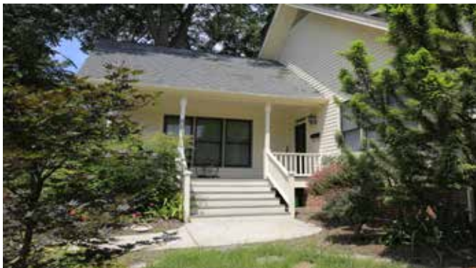
Side facing entrance on Latham St
