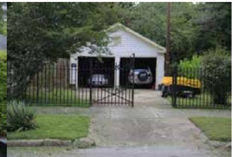
414 N. Bloodworth Street—two car garage and concrete drive adjacent to house, facing Bloodworth St.
