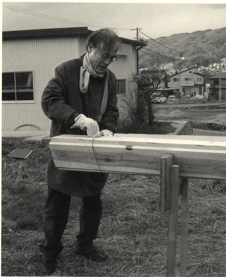
Fujimori preparing the cedar boards to be charred (above). The process reveals Fujimori's ritualistic approach to his buildings (opposite).
