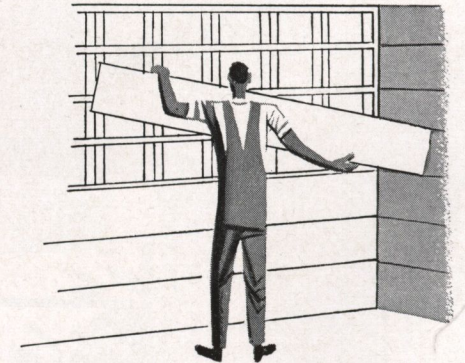
For horizontal application of Finish Plank, furring strips are applied behind all joints.
